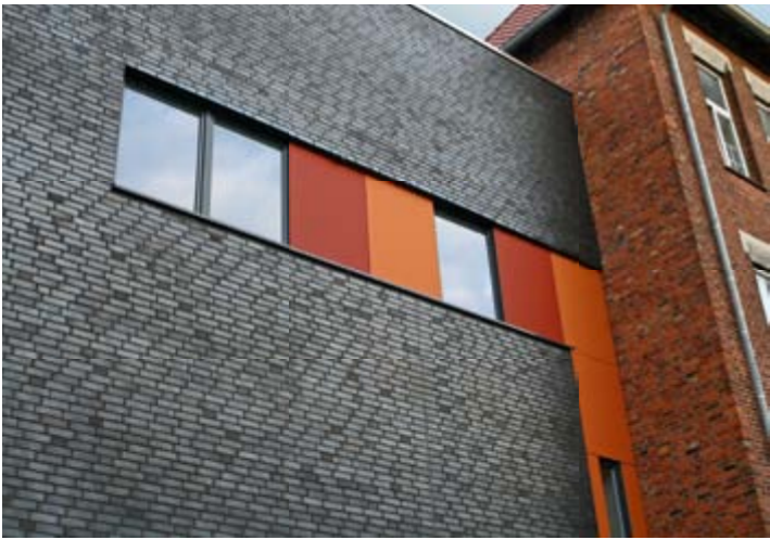
On the outside modern Röben clinker brick Cambridge, on the inside the indestructible and extremely resilient Röben fine stoneware VIGRANIT.
