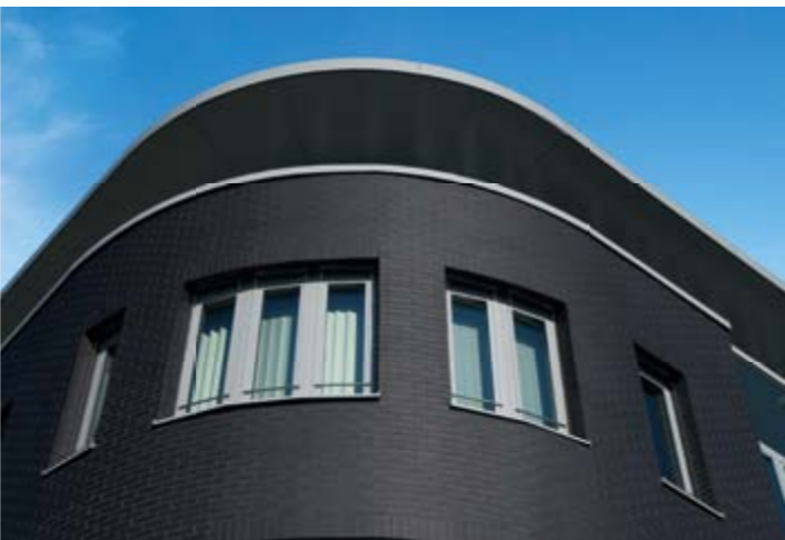
Clean curves with Röben ceramic clinker brick strip tiles. A modern thermal insulate composite system is concealed underneath.
