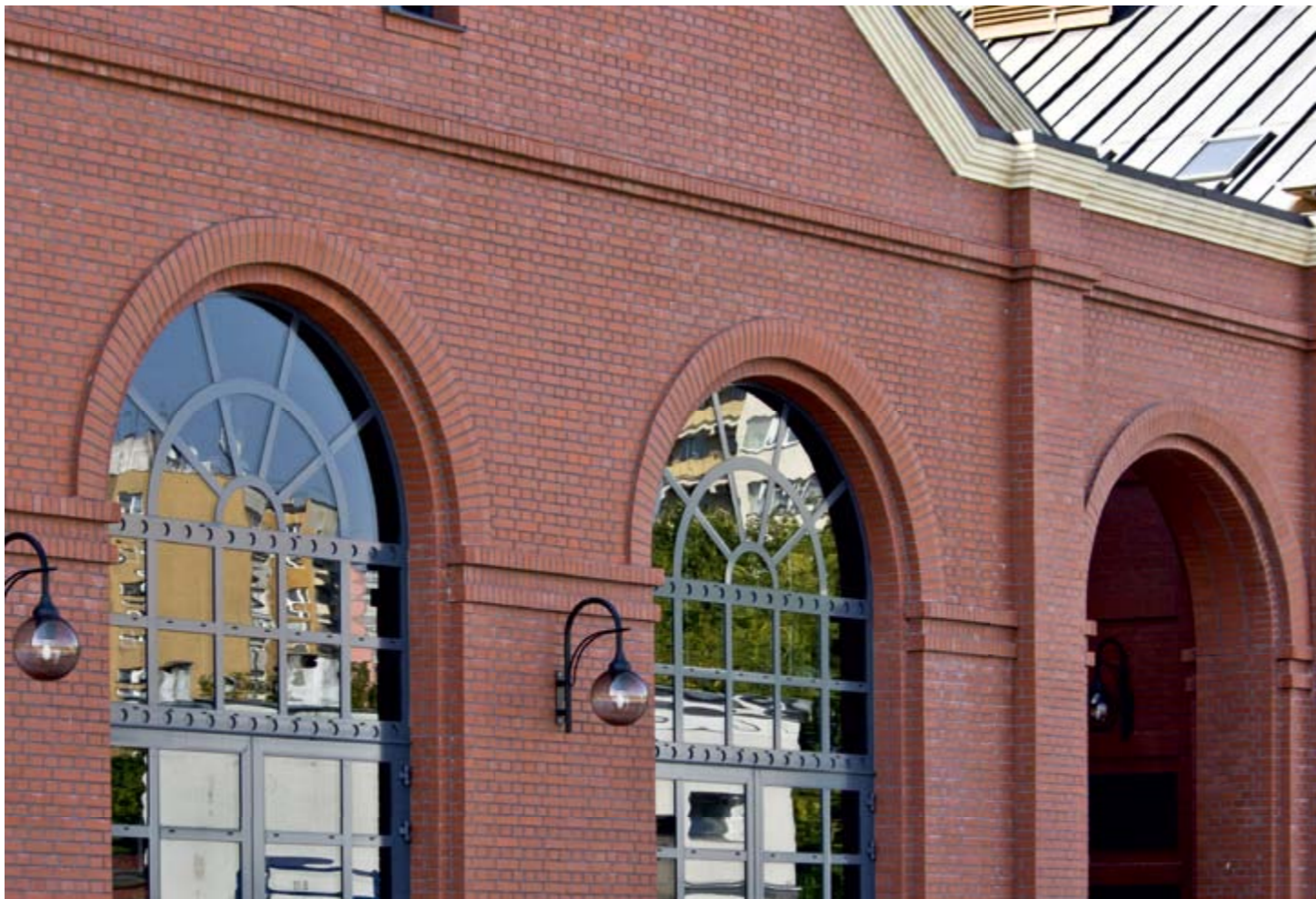
At the request of the architects, around 1,600 arch bricks were fired to create the arcade arches.
