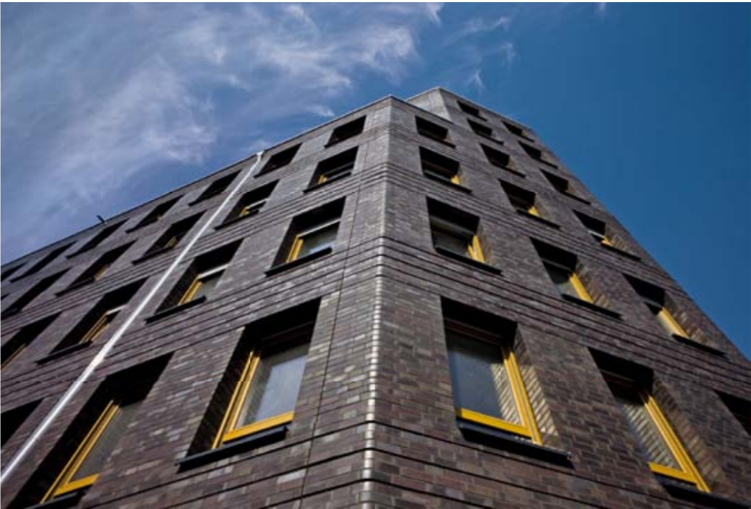
Above: All lintels were Röben prefabricated elements. Below: The building's corners with angles of 45° were designed with Röben shaped bricks.
